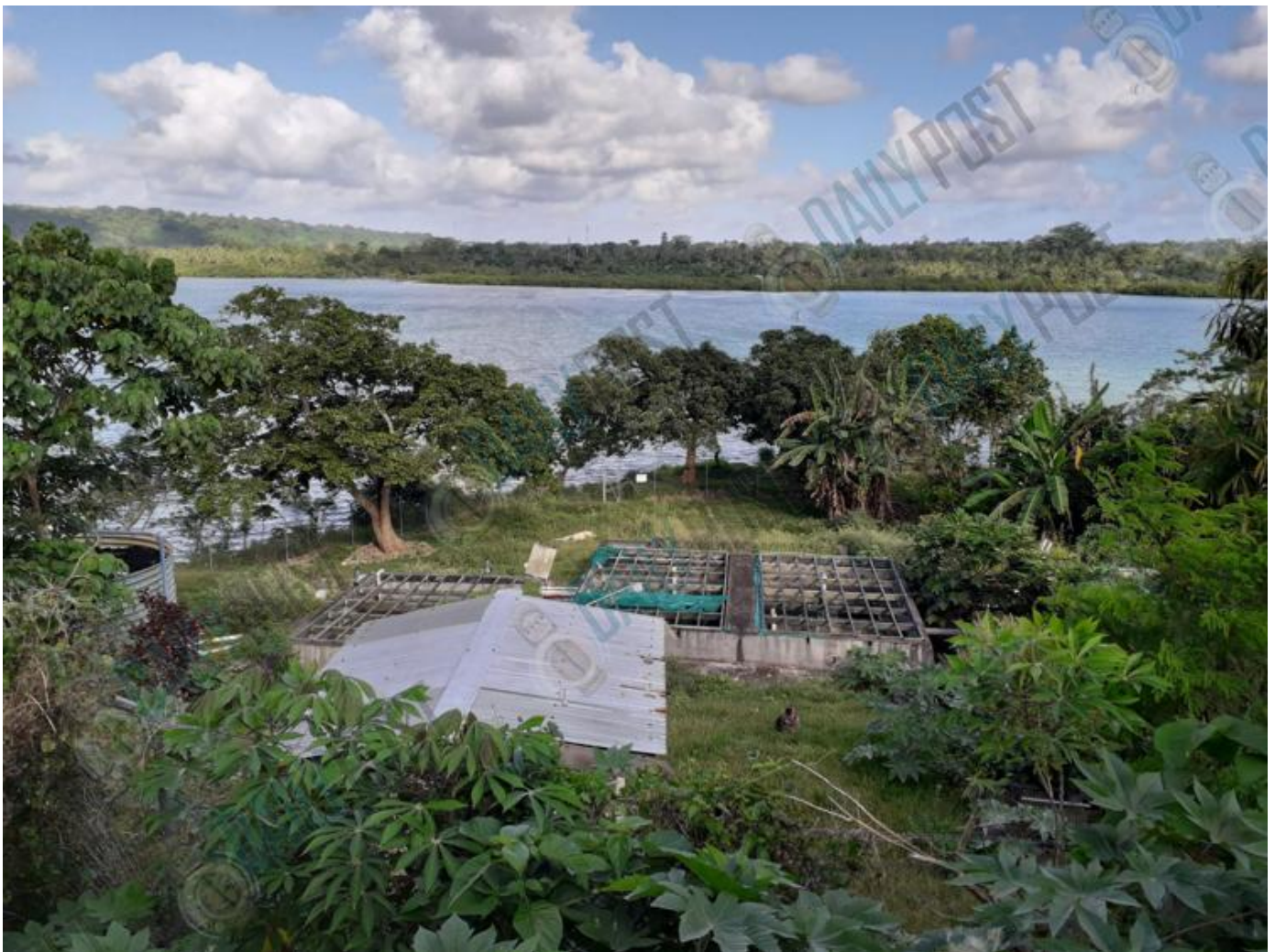
Vila Central Hospital's current sewage system
