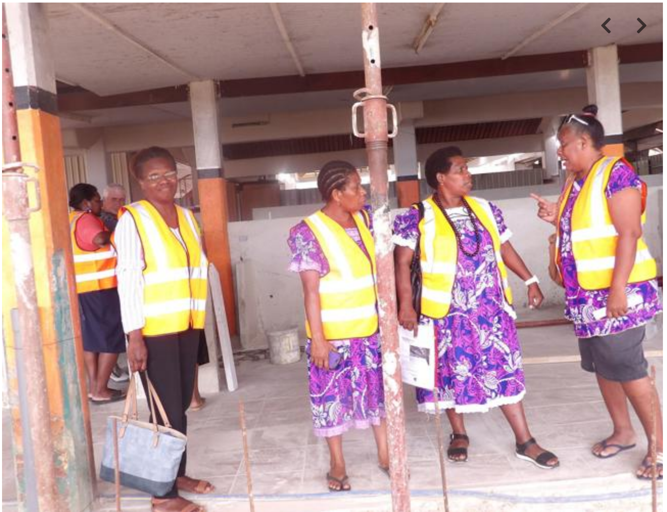
Representatives of stakeholders checking renovation in Restaurant Wing
