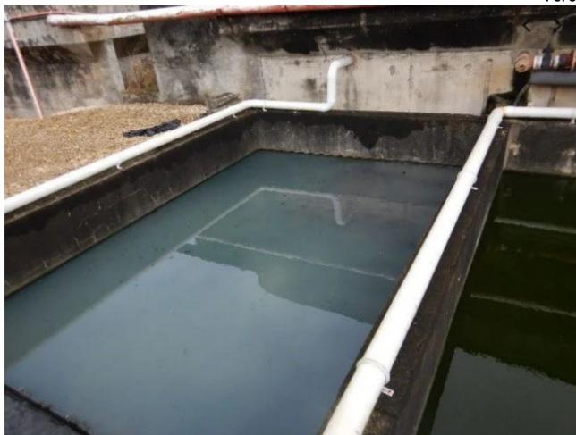
The Chlorination Tank.With high turbidity, chlorination is not effective, according to the water quality report. Photos: Do<sup>1</sup>
