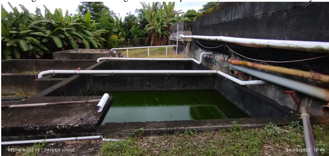
Stagnant water with algal growth, deteriorated pipework, tank wall's structure appears good
