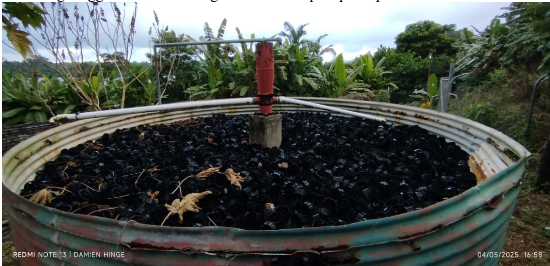
Trickling filter – Condition rating: Poor. Non-operational, been out of service for years
