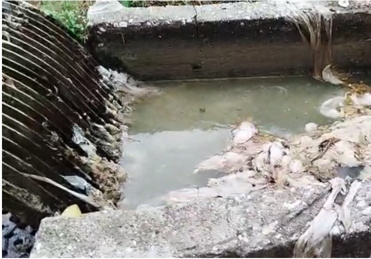
Screening clogged – no visible signs of routine upkeep or operator attendance
